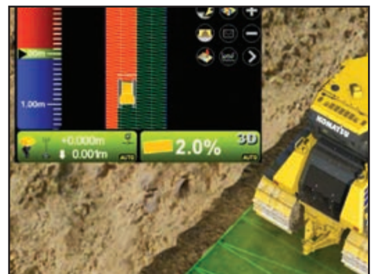
Surface track mapping: cab top GNSS antenna collects accurate “as-built” surface data. It measures actual elevations, as the machine continuously tracks in operation.
