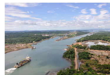
Dock deepening & extension
