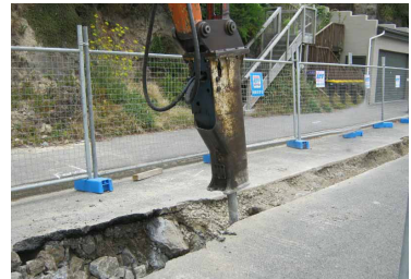
Trenching, pit building, ground excavation
