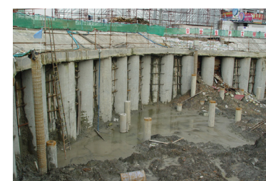
Foundation pile driving
