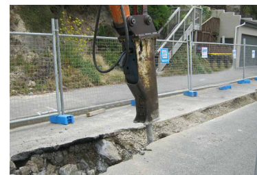
Trenching, pit building, ground excavation
