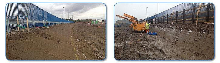
The top 21 degree slope was cut using traditional site engineering methods utilising profile boards, batter rails, string line and a measuring tape making this labour intensive and a relatively slow process. Lots of options were considered on how L&C would control the line & level during the cutting of the 65 degree slope. L&C tried using templates, rotating lasers, profile boards, batter rails and a robotic total station.
