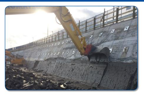
A surveyor from Marubeni-Komatsu came to site with the machine to set up the GPS system and load the 3D model into the machine's computer. A fully trained Komatsu demonstration driver also came and gave L&C's excavator operator a short tutorial on how to use the computer and the controls. Soon the operator was cutting the 65 degree slope with ease and without the need for a banksman constantly checking the accuracy.
