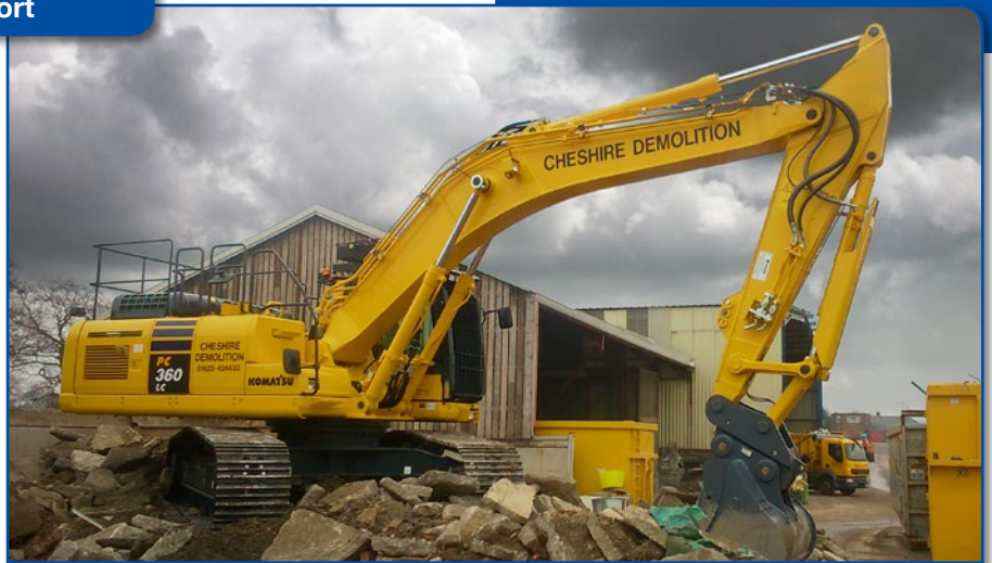
Cheshire Demolition's PC360LC hard at work on site
